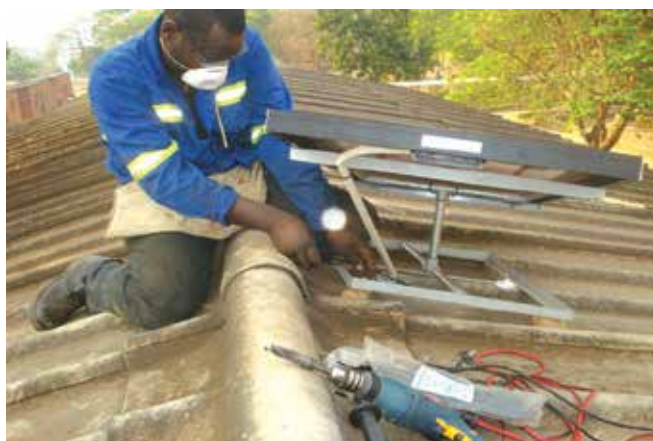
Technician installing solar PV at Kanyanga RHC
